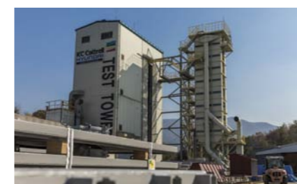
Bag filter test tower
