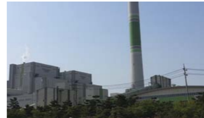
Yoengheoung Thermal Power Plant
