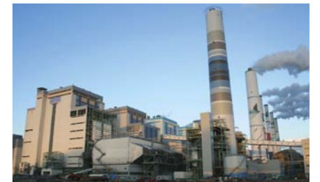
Taean Thermal Power Plant
