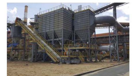
POSCO E&C CSP Steel Plant Coke Plant
