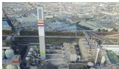
Daegu Dyeing Complex Cogeneration Power Plant
