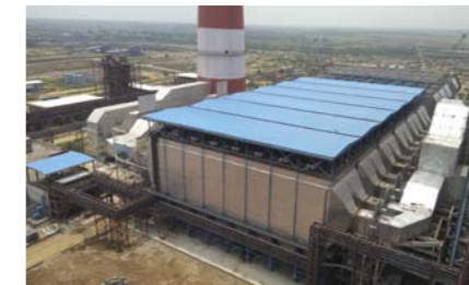
NTPC Meja Thermal Power Plant
