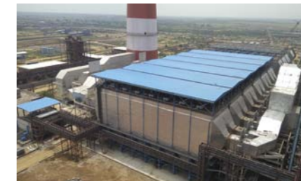
NTPC Meja Thermal Power Plant
