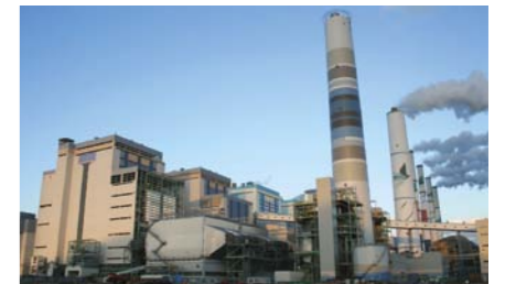
Taean Thermal Power Plant
