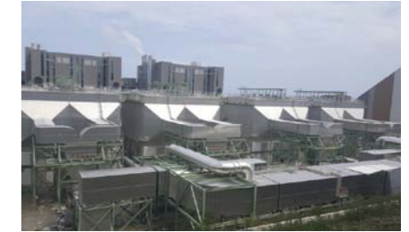
Samcheok Green Thermal Power Plant
