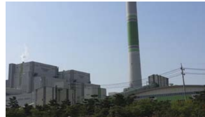
Yoengheoung Thermal Power Plant
