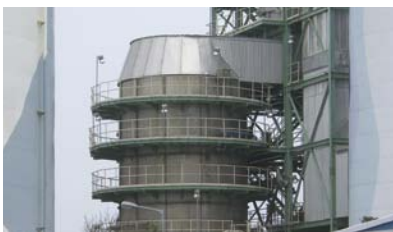
Jeju Internal Combustion Plant
