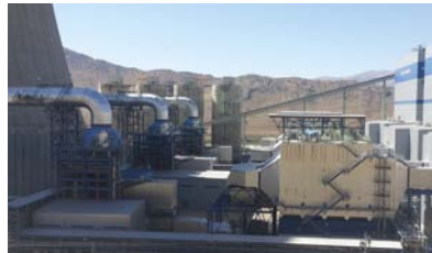
Tufanbeyli Thermal Power Plant
