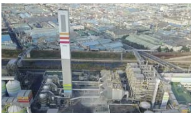
Daegu Dyeing Complex Cogeneration Power Plant
