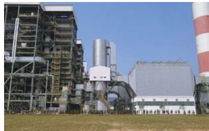
Saemangeum Thermal Power Plant
