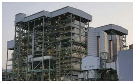
Saemangeum Power Plant
