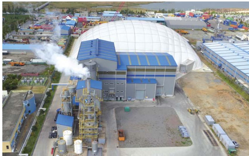
KC Enviro Services(Yeosu-Hwachang) : Industrial Waste Treatment, Fluidized Bed Combustion(FBC), Steam Supply and Sanitary Landfill
