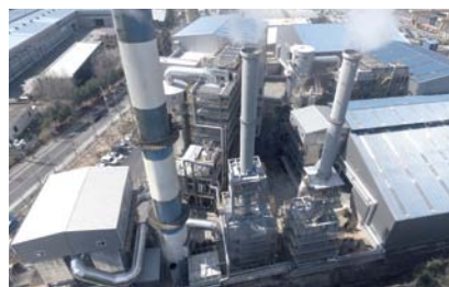
Changwon Enerotec : Industrial Waste Treatment, Stoker, SRF Boiler, SRF Manufacturing, Steam Supply and 2.75MW Power Plant
